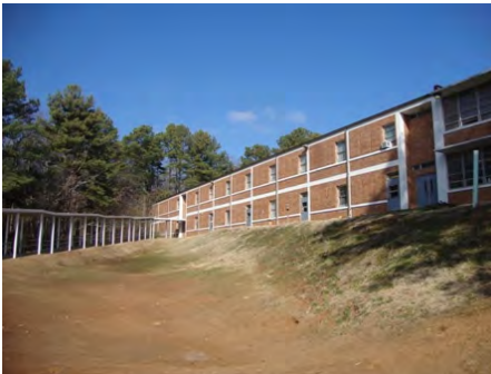
11-Feb-2011 South Elevation
