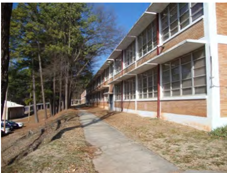
11-Feb-2011 South Elevation
