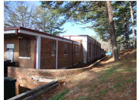
11-Feb-2011 North Elevation
