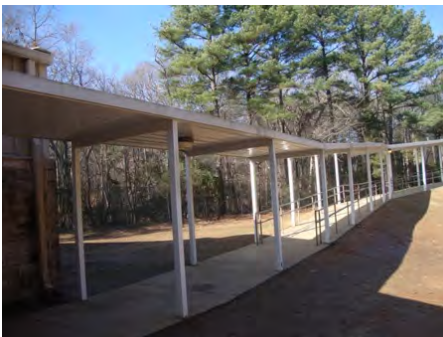
11-Feb-2011 North Elevation
