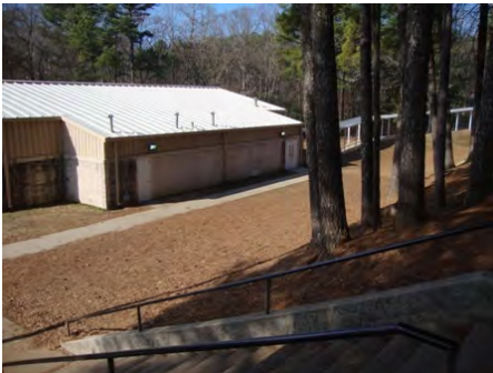
11-Feb-2011 North Elevation
