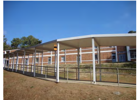
11-Feb-2011 South Elevation
