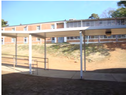
11-Feb-2011 South Elevation
