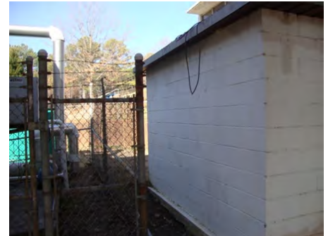
11-Feb-2011 South Elevation
