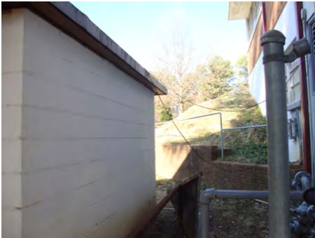
11-Feb-2011 North Elevation
