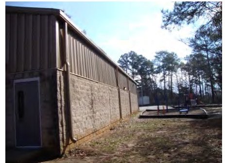
11-Feb-2011 South Elevation
