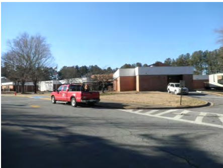
08-Feb-2011 North Elevation
