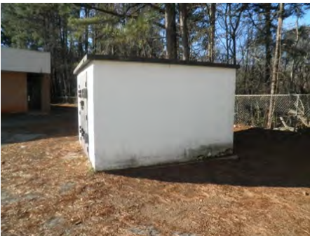
08-Feb-2011 North Elevation
