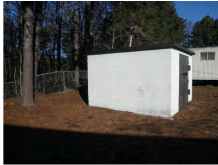
08-Feb-2011 South Elevation
