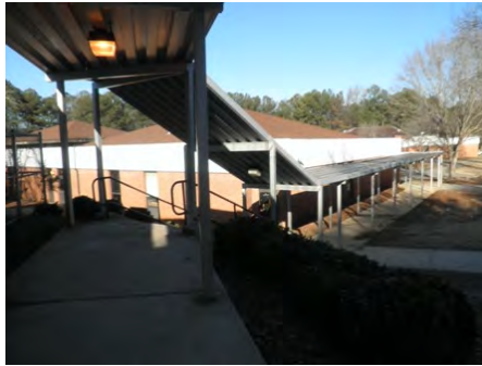
08-Feb-2011 South Elevation
