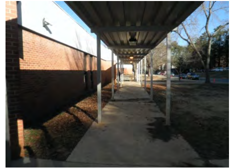
08-Feb-2011 North Elevation
