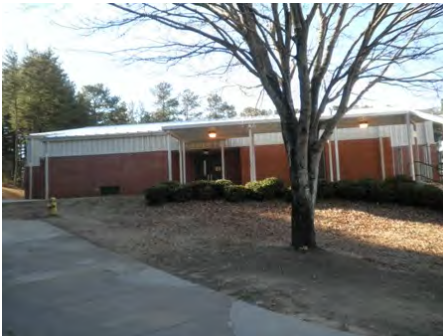
08-Feb-2011 North Elevation
