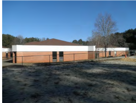
08-Feb-2011 South Elevation
