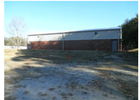
08-Feb-2011 South Elevation
