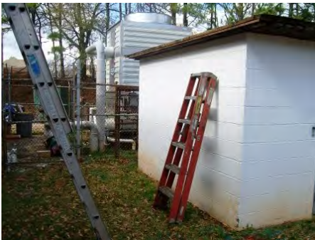
25-Feb-2011 South Elevation
