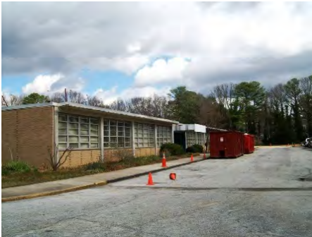
25-Feb-2011 South Elevation
