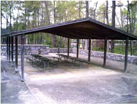
25-Feb-2011 North Elevation
