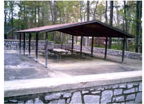
25-Feb-2011 South Elevation
