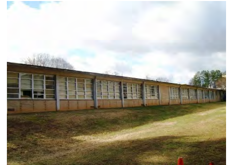
25-Feb-2011 North Elevation
