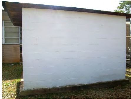
25-Feb-2011 North Elevation
