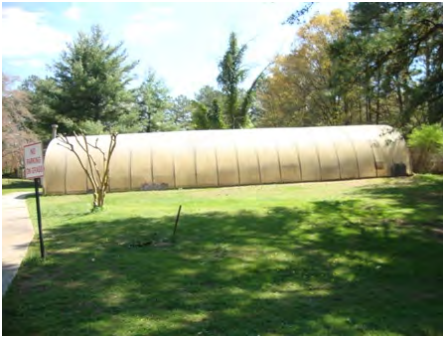
24-Mar-2011 North Elevation
