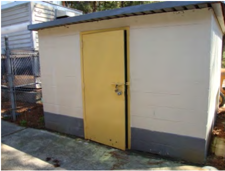
24-Mar-2011 North Elevation
