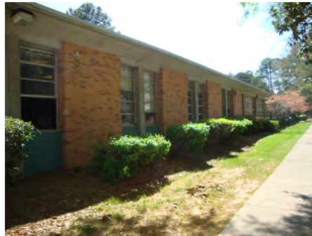
24-Mar-2011 North Elevation
