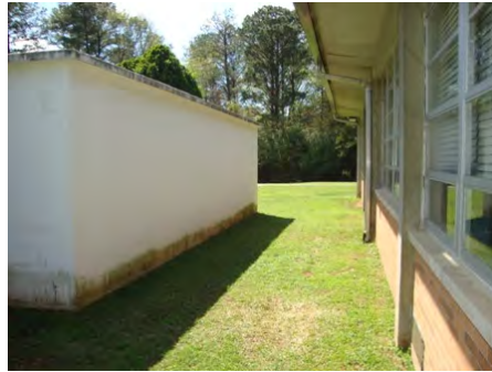
24-Mar-2011 North Elevation
