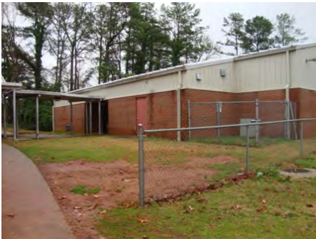
09-Mar-2011 North Elevation
