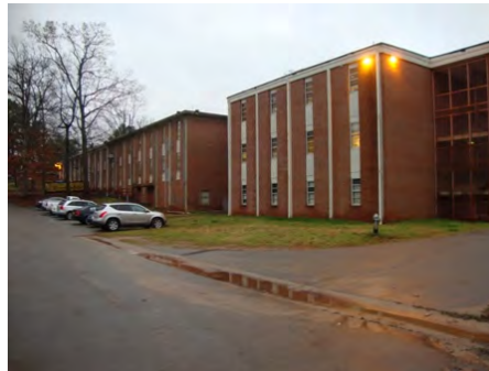
09-Mar-2011 Southwest Elevation
