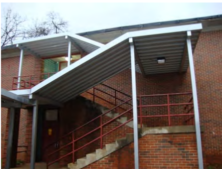
09-Mar-2011 North Elevation
