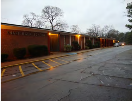
09-Mar-2011 North Elevation
