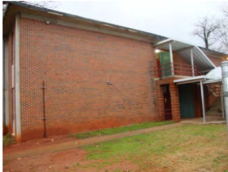
09-Mar-2011 Northeast Elevation
