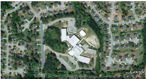
28-Dec-2010 Aerial Image of Shadow Rock Elementary School
