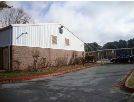
10-Feb-2011 South Elevation
