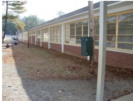
10-Feb-2011 North Elevation
