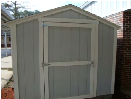
10-Feb-2011 North Elevation
