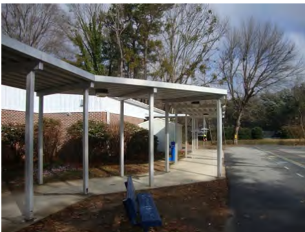
10-Feb-2011 South Elevation
