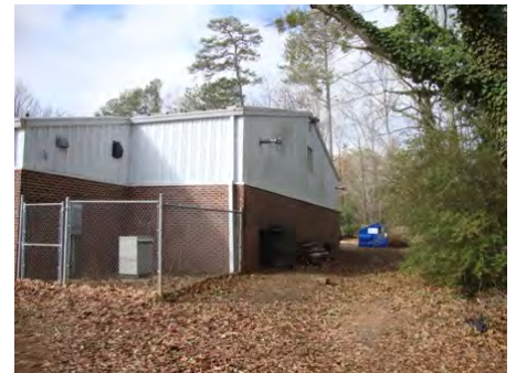
10-Feb-2011 North Elevation
