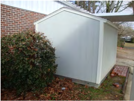
10-Feb-2011 South Elevation
