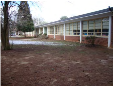
10-Feb-2011 South Elevation
