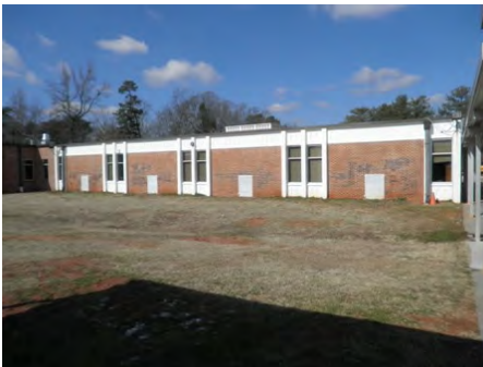
10-Feb-2011 South Elevation
