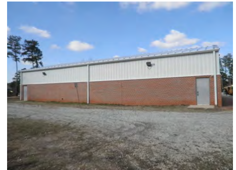
10-Feb-2011 South Elevation
