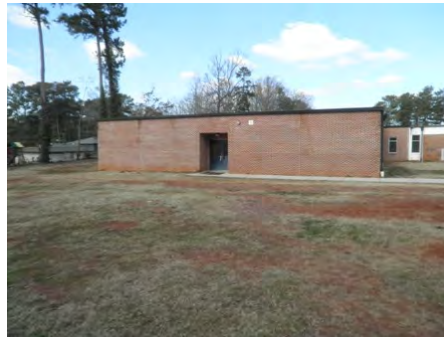
10-Feb-2011 South Elevation
