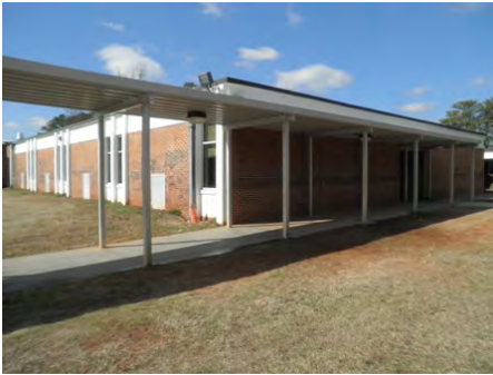
10-Feb-2011 East Elevation
