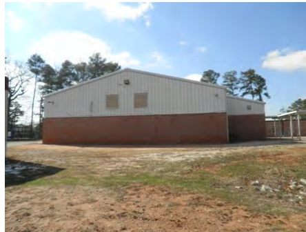
10-Feb-2011 East Elevation
