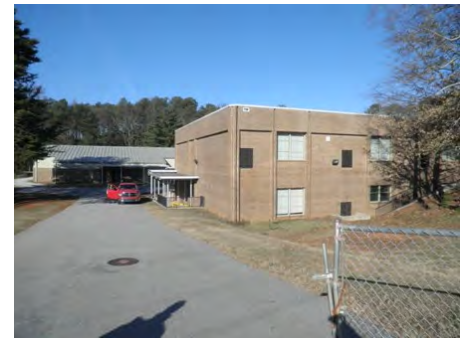
09-Dec-2010 Southwest Elevation
