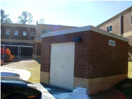
06-Dec-2010 Northeast Elevation
