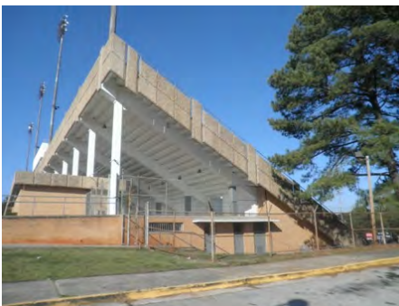
23-Feb-2011 South Elevation
