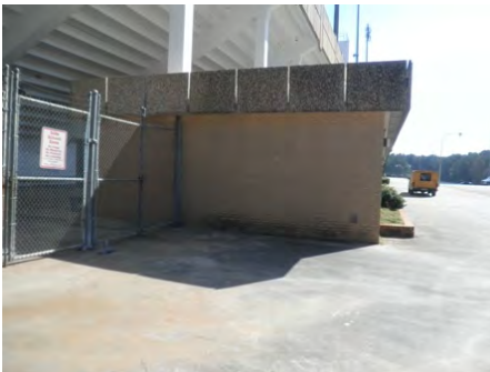
23-Feb-2011 North Elevation
