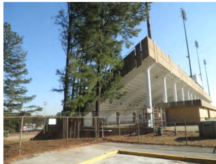
23-Feb-2011 North Elevation
