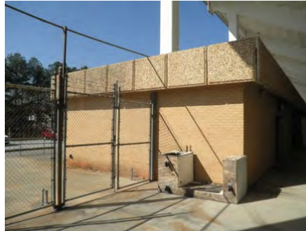
23-Feb-2011 South Elevation
