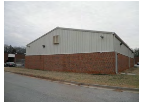
07-Feb-2011 South Elevation
