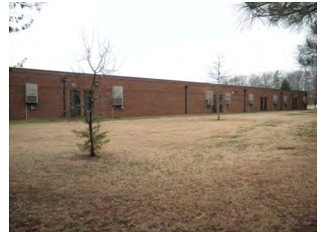
07-Feb-2011 North Elevation
