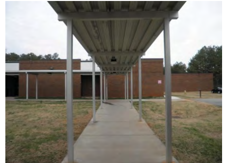
07-Feb-2011 South Elevation
