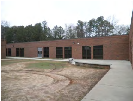
07-Feb-2011 South Elevation
