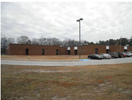
07-Feb-2011 South Elevation
