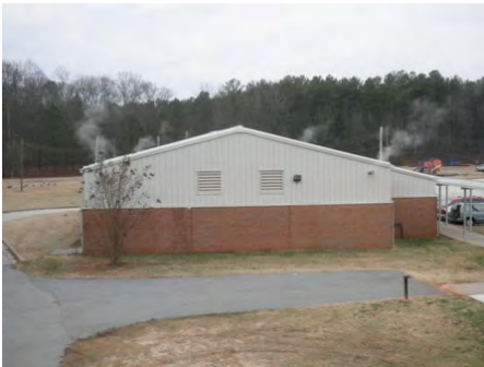
07-Feb-2011 North Elevation
