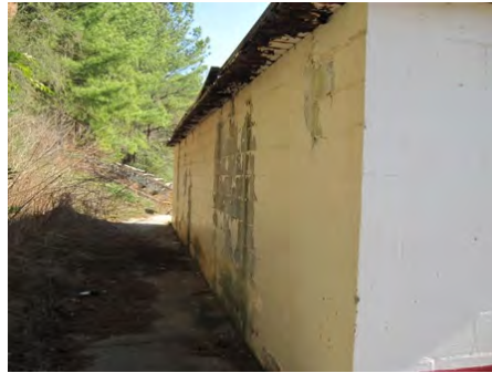
23-Feb-2011 North Elevation
