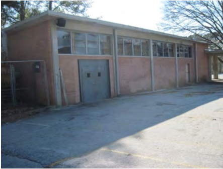
23-Feb-2011 North Elevation
