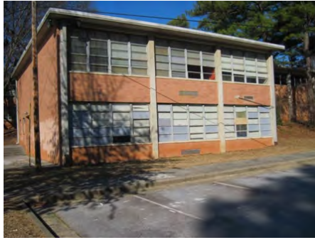
23-Feb-2011 South Elevation
