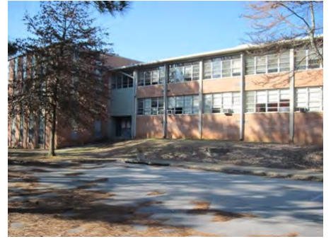
23-Feb-2011 South Elevation
