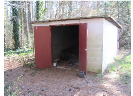
23-Feb-2011 North Elevation
