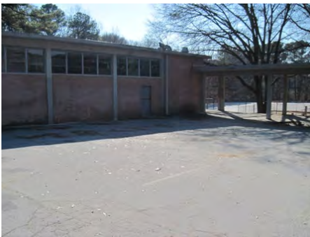
23-Feb-2011 Southeast Elevation
