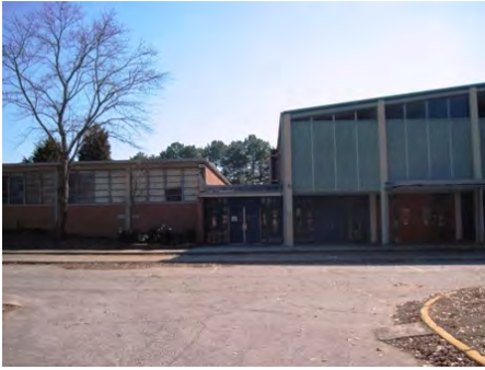
23-Feb-2011 North Elevation
