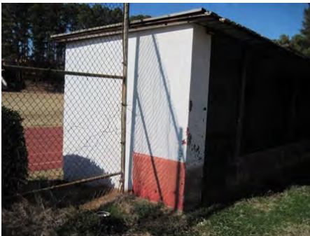
23-Feb-2011 South Elevation
