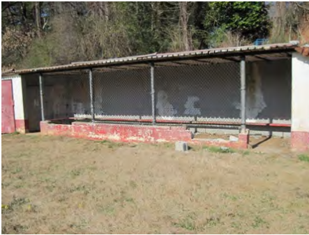
23-Feb-2011 South Elevation
