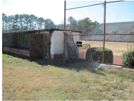
23-Feb-2011 North Elevation
