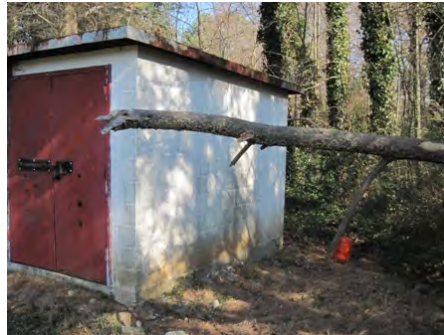
23-Feb-2011 South Elevation
