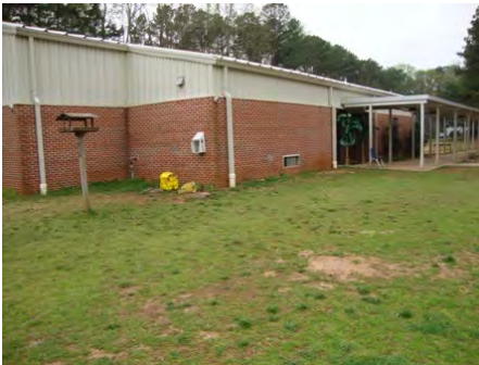
21-Mar-2011 North Elevation
