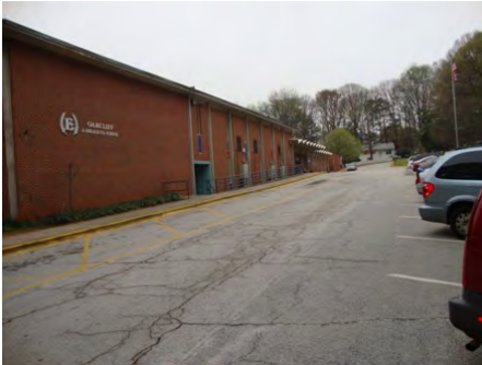
21-Mar-2011 North Elevation
