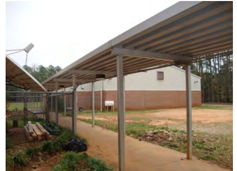
21-Mar-2011 North Elevation
