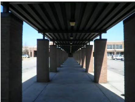
22-Feb-2011 South Elevation
