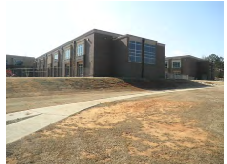
22-Feb-2011 North Elevation
