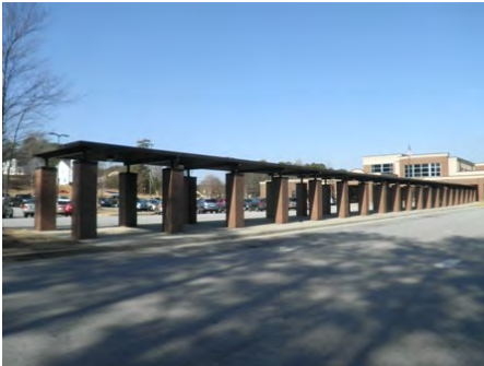
22-Feb-2011 Southeast Elevation
