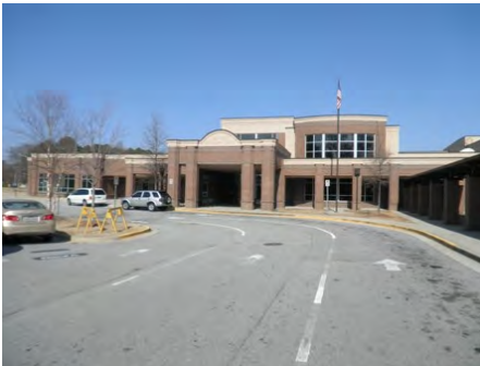
22-Feb-2011 South Elevation
