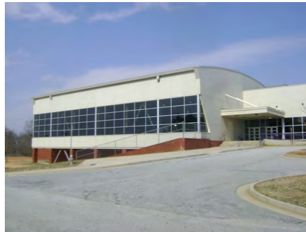
24-Feb-2011 South Elevation
