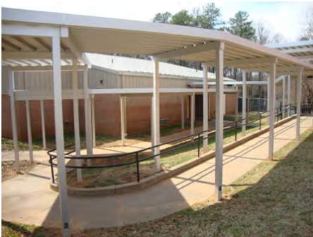
24-Feb-2011 North Elevation
