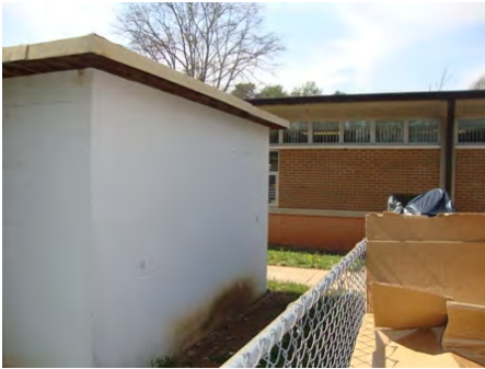
24-Feb-2011 North Elevation
