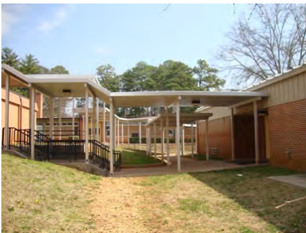
24-Feb-2011 Southwest Elevation
