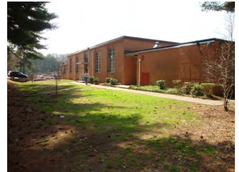
24-Feb-2011 South Elevation
