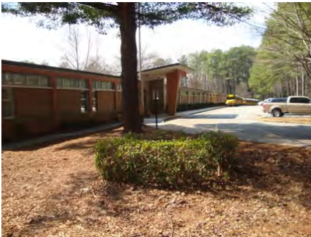
24-Feb-2011 North Elevation
