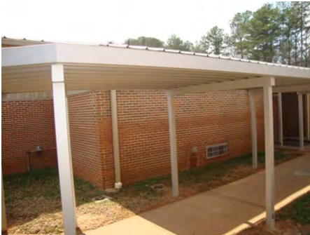
24-Feb-2011 North Elevation
