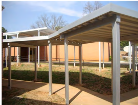
24-Feb-2011 South Elevation
