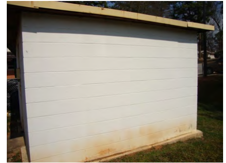
24-Feb-2011 South Elevation
