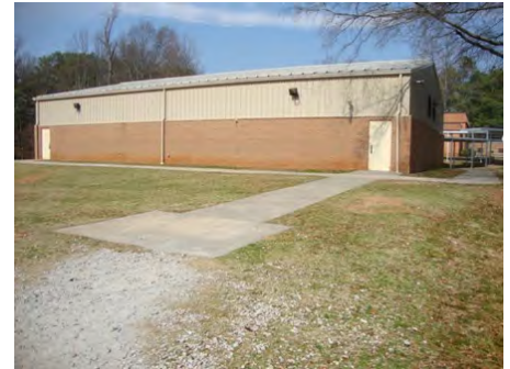
24-Feb-2011 South Elevation
