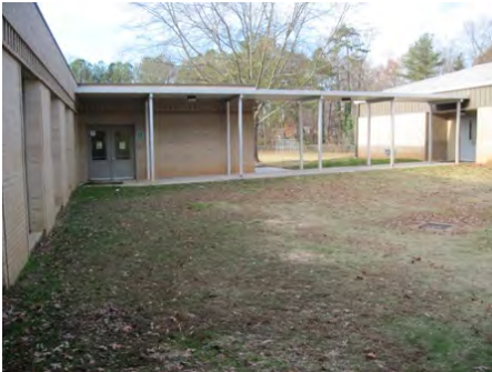
06-Dec-2010 Northeast Elevation
