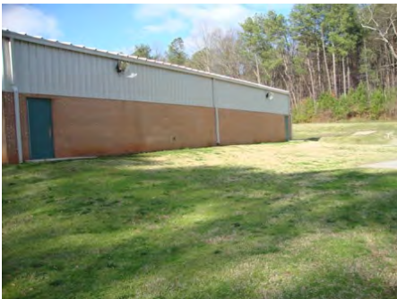
11-Mar-2011 North Elevation
