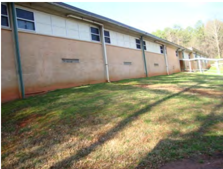
11-Mar-2011 North Elevation
