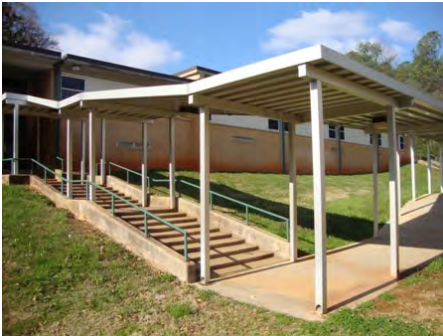
11-Mar-2011 Northeast Elevation
