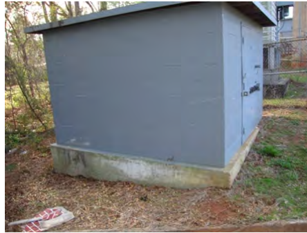
11-Mar-2011 North Elevation
