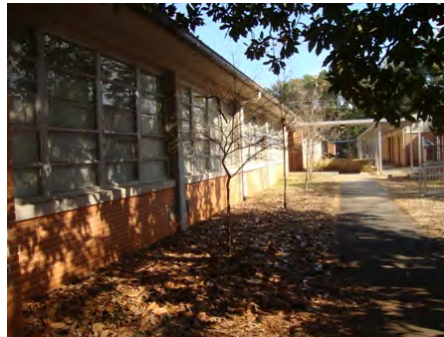
11-Feb-2011 South Elevation
