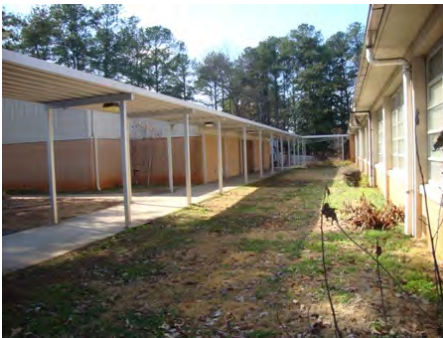
11-Feb-2011 North Elevation
