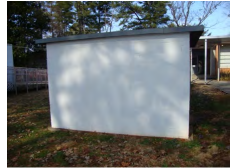
11-Feb-2011 South Elevation
