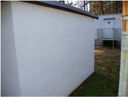
11-Feb-2011 North Elevation
