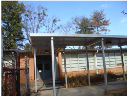
11-Feb-2011 South Elevation
