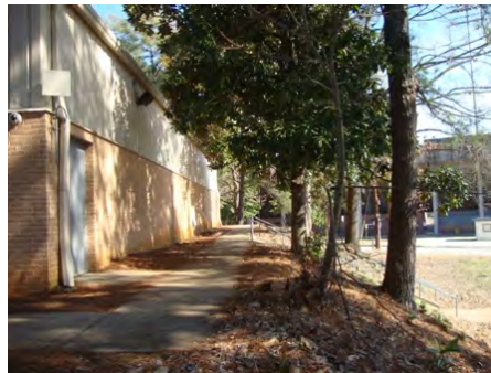
11-Feb-2011 South Elevation
