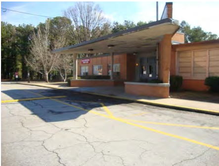
11-Feb-2011 North Elevation
