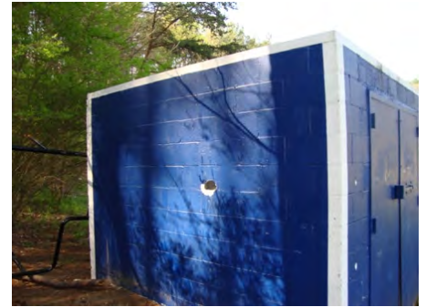
23-Mar-2011 North Elevation
