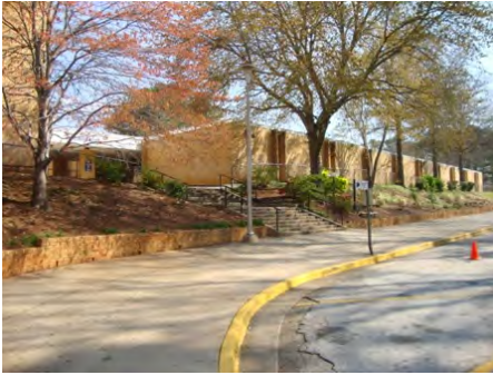
23-Mar-2011 North Elevation
