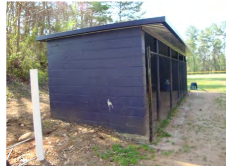
23-Mar-2011 North Elevation
