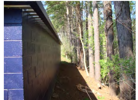
23-Mar-2011 North Elevation
