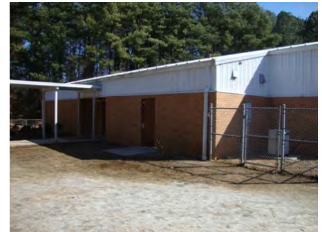
08-Feb-2011 South Elevation
