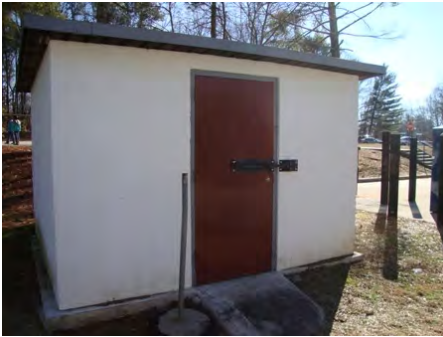
08-Feb-2011 South Elevation
