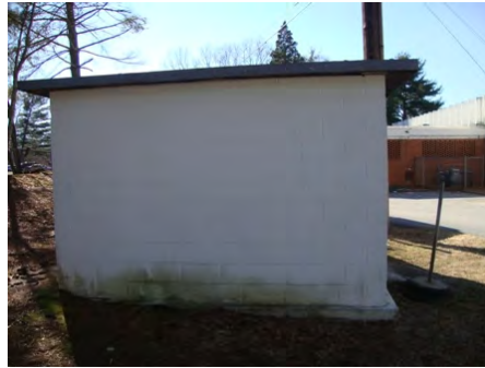
08-Feb-2011 East Elevation
