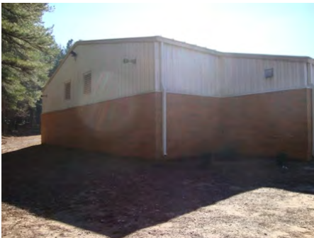
08-Feb-2011 East Elevation
