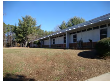
08-Feb-2011 South Elevation
