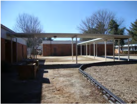
08-Feb-2011 East Elevation
