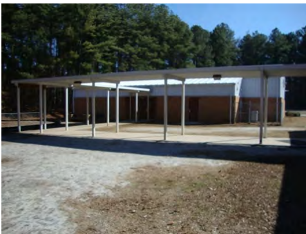
08-Feb-2011 South Elevation
