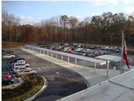
01-Dec-2010 Southwest Elevation
