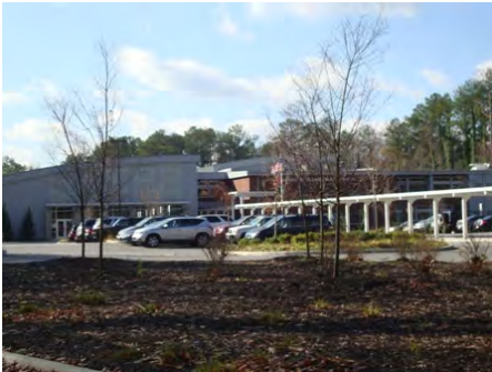
01-Dec-2010 Northeast Elevation
