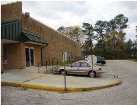
23-Mar-2011 North Elevation
