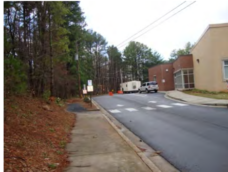
25-Feb-2011 East Elevation
