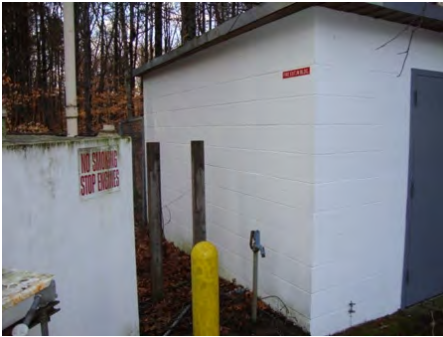
25-Feb-2011 North Elevation
