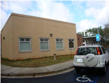
25-Feb-2011 North Elevation
