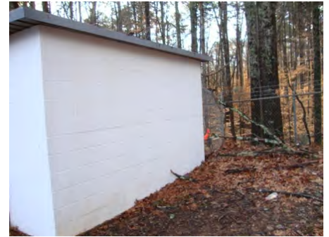
25-Feb-2011 South Elevation
