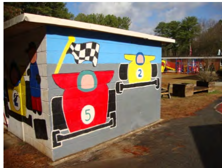
25-Feb-2011 East Elevation
