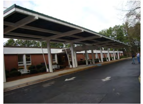
25-Feb-2011 North Elevation
