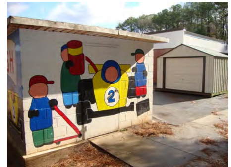
25-Feb-2011 South Elevation
