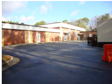
25-Feb-2011 East Elevation
