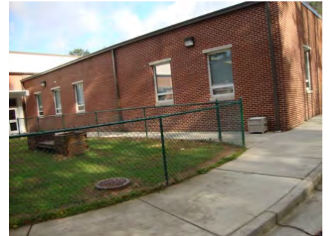
25-Feb-2011 South Elevation
