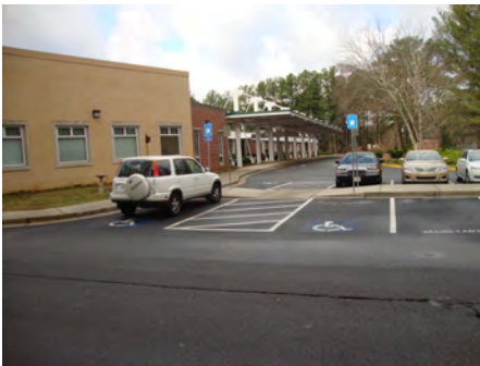
25-Feb-2011 North Elevation
