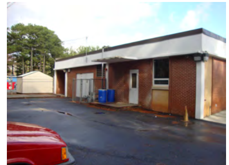
25-Feb-2011 South Elevation
