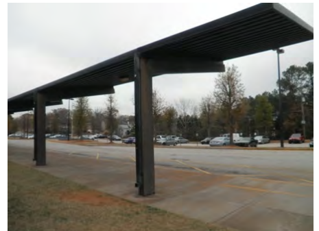
08-Dec-2010 Southwest Elevation
