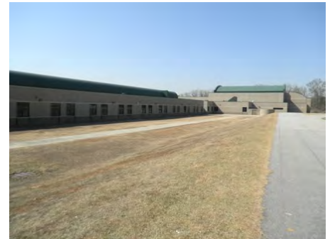
23-Feb-2011 North Elevation
