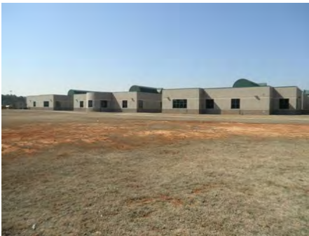
23-Feb-2011 East Elevation
