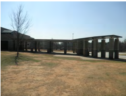
23-Feb-2011 North Elevation
