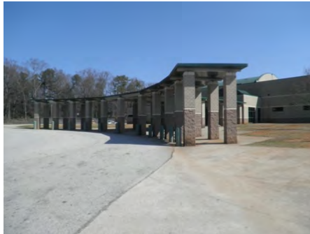
23-Feb-2011 Southwest Elevation
