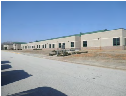
23-Feb-2011 South Elevation
