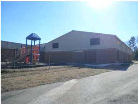
22-Feb-2011 East Elevation
