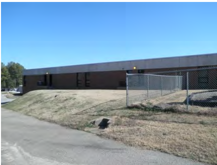
22-Feb-2011 North Elevation
