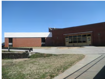
22-Feb-2011 North Elevation
