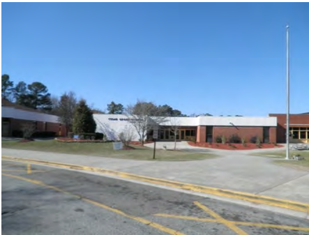
22-Feb-2011 South Elevation
