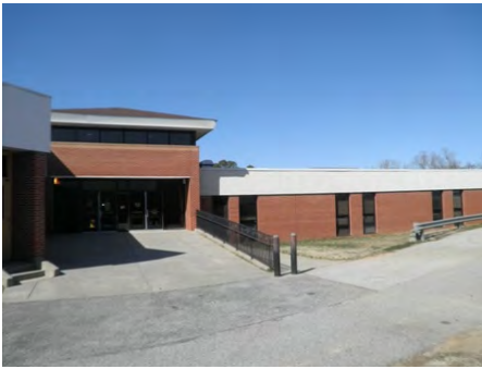
22-Feb-2011 South Elevation
