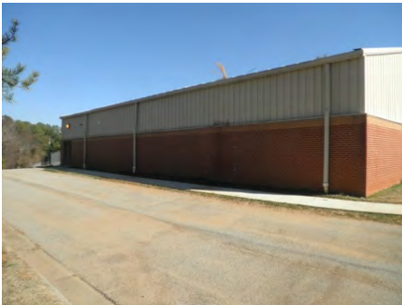
22-Feb-2011 North Elevation
