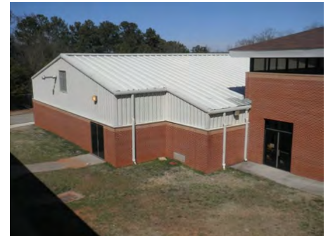
22-Feb-2011 South Elevation
