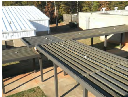
09-Dec-2010 Northeast Elevation
