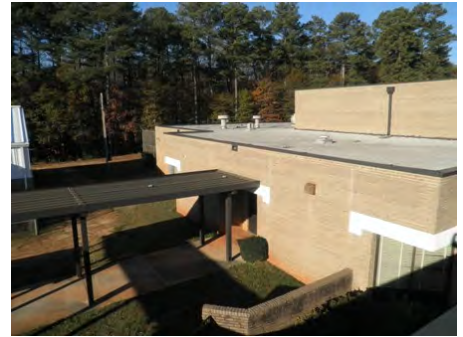
09-Dec-2010 Northeast Elevation
