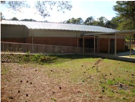
25-Mar-2011 North Elevation
