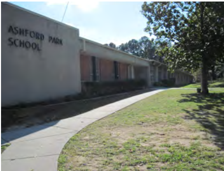
25-Mar-2011 North Elevation
