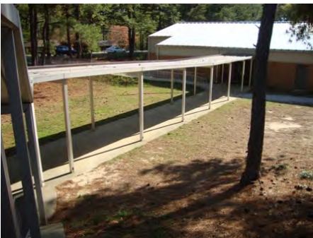
25-Mar-2011 North Elevation
