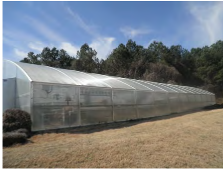
08-Mar-2011 North Elevation
