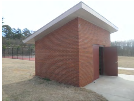
08-Mar-2011 North Elevation
