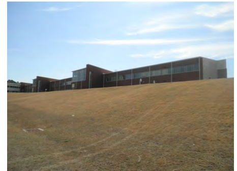
08-Mar-2011 North Elevation
