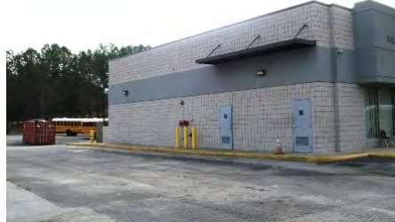
24-Feb-2011 South Elevation
