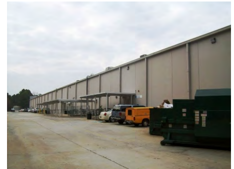
24-Feb-2011 East Elevation
