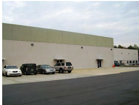
24-Feb-2011 South Elevation
