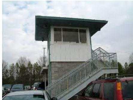
24-Feb-2011 South Elevation
