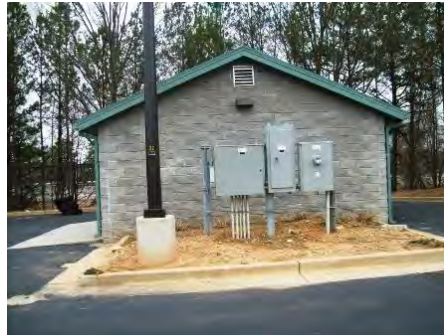
24-Feb-2011 South Elevation
