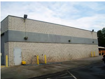
24-Feb-2011 North Elevation
