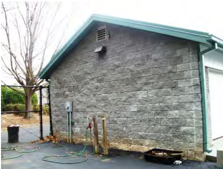
24-Feb-2011 North Elevation
