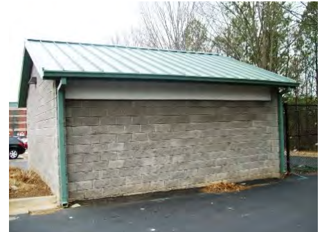
24-Feb-2011 East Elevation
