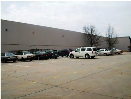
24-Feb-2011 North Elevation
