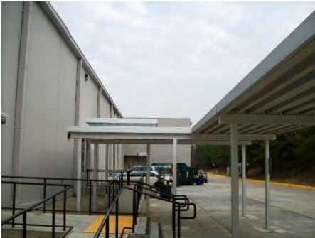
24-Feb-2011 South Elevation
