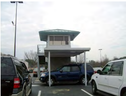
24-Feb-2011 North Elevation
