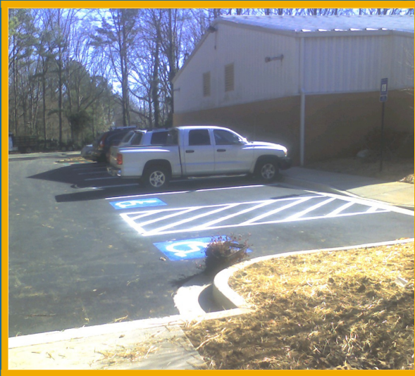
Montgomery Elementary - Paving ▼
