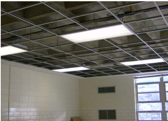
Shamrock MS Classroom Ceiling Grid – Area 4
