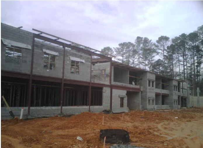
Dunwoody Area ES Unfinished Exterior View of Classrooms
