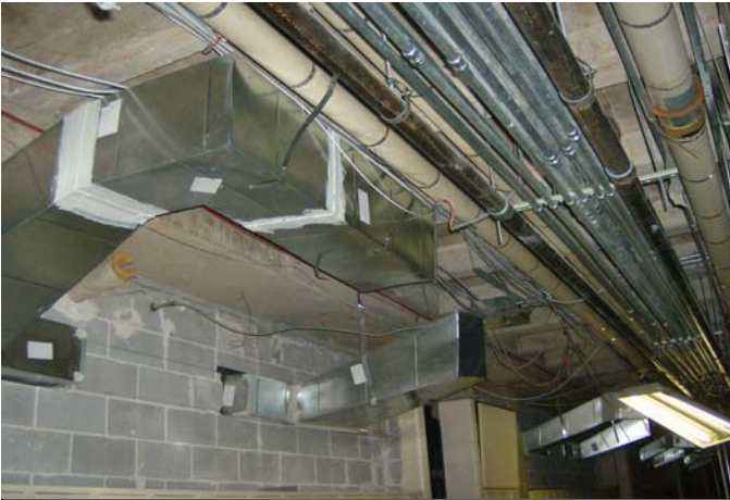
Sequoyah MS Ductwork Installation in Corridor
