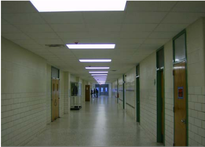
Shamrock MS Completed Corridor– Area 7
