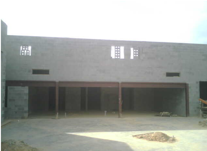
Dunwoody Area ES Unfinished Interior View of Cafetorium
