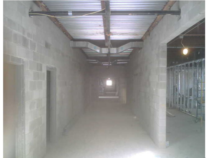
Dunwoody Area ES View of Unfinished Corridor
