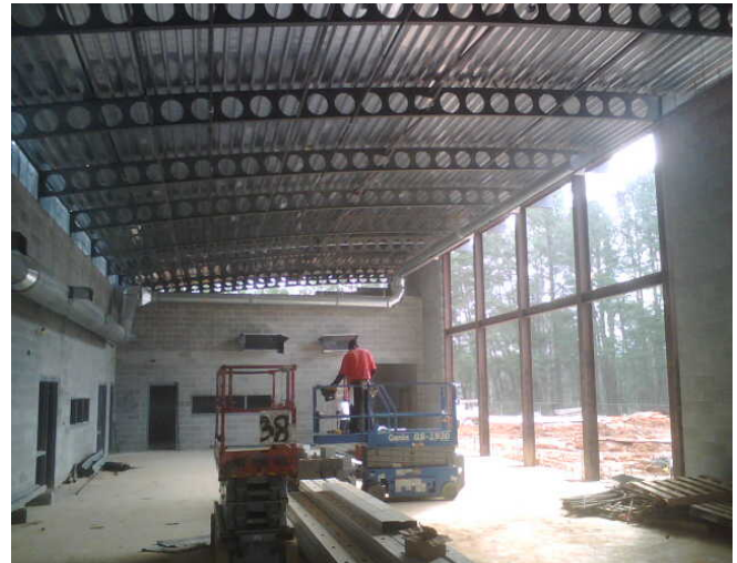
Dunwoody Area ES Unfinished Interior View of Media Center
