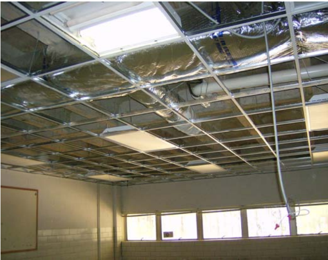
Sequoyah MS Classroom Ceiling Grid Installation
