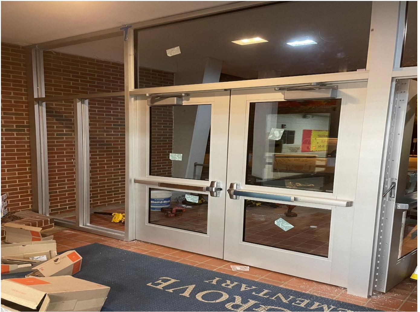
Exterior Storefront Installation
