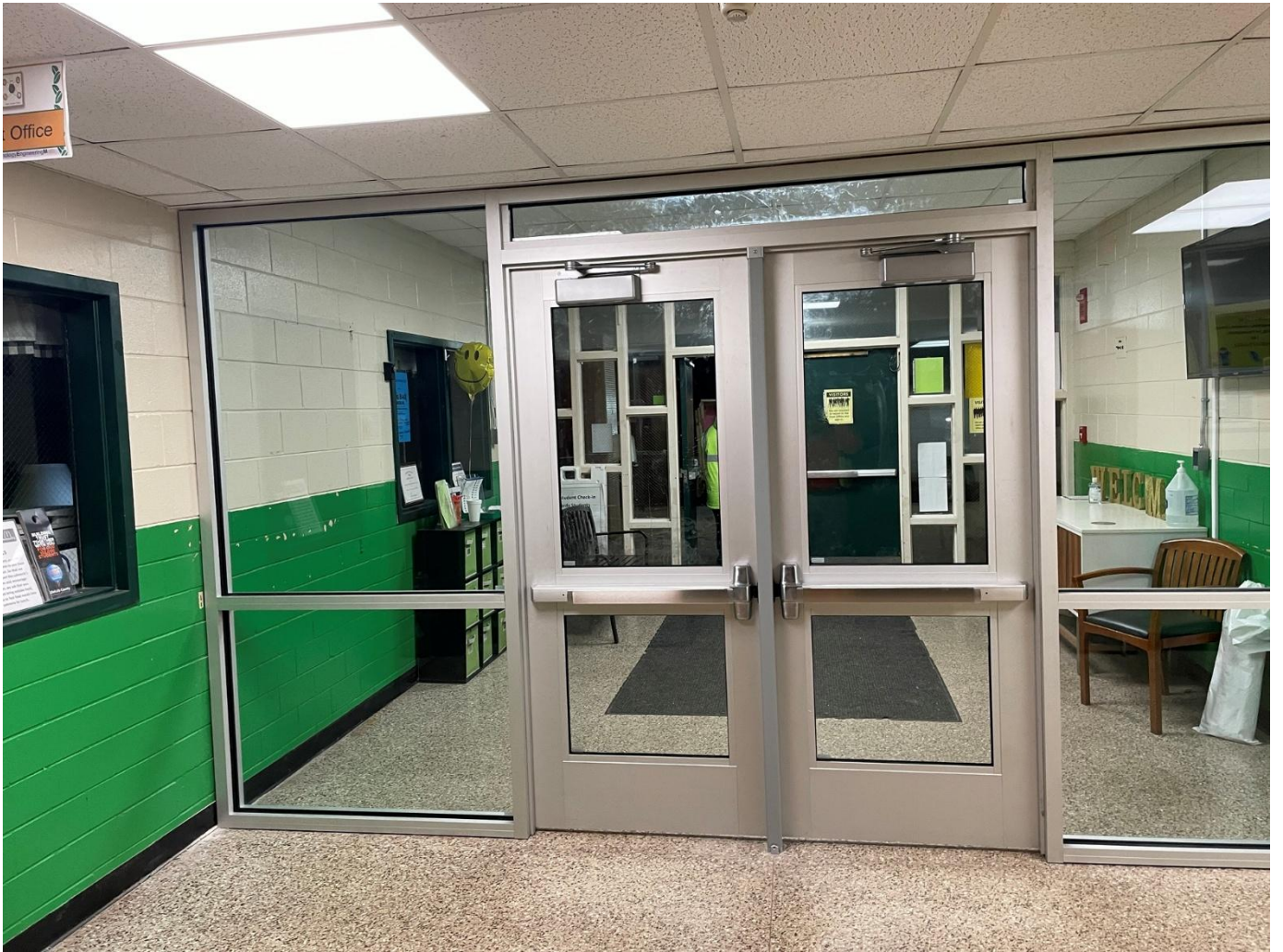
Interior Security Vestibule Installation.
