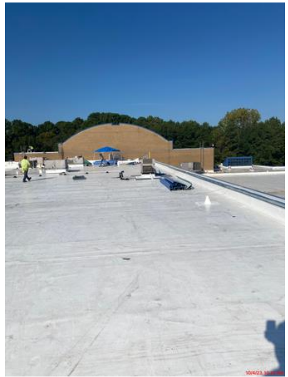
Installing Metal Trim
