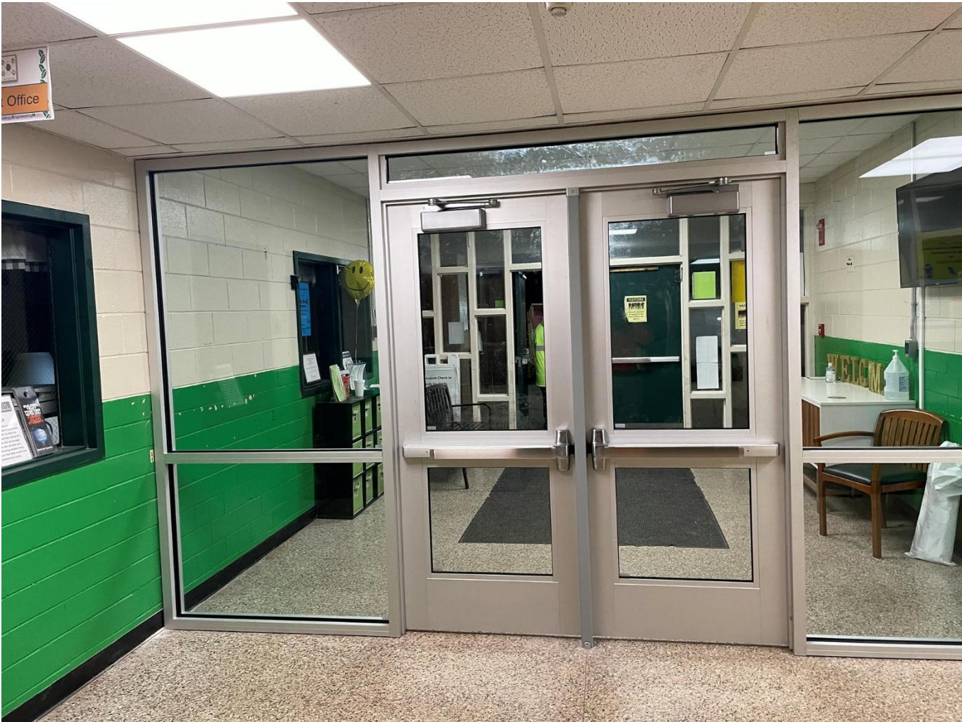
Interior Security Vestibule Installation.
