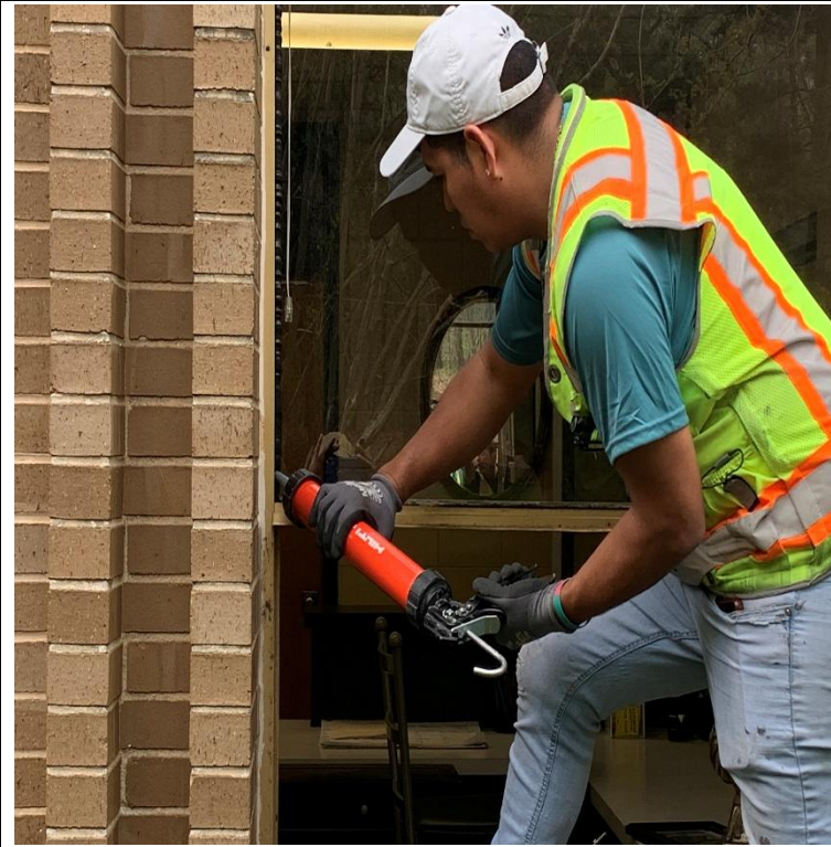
Tampered Glass Window Installation
