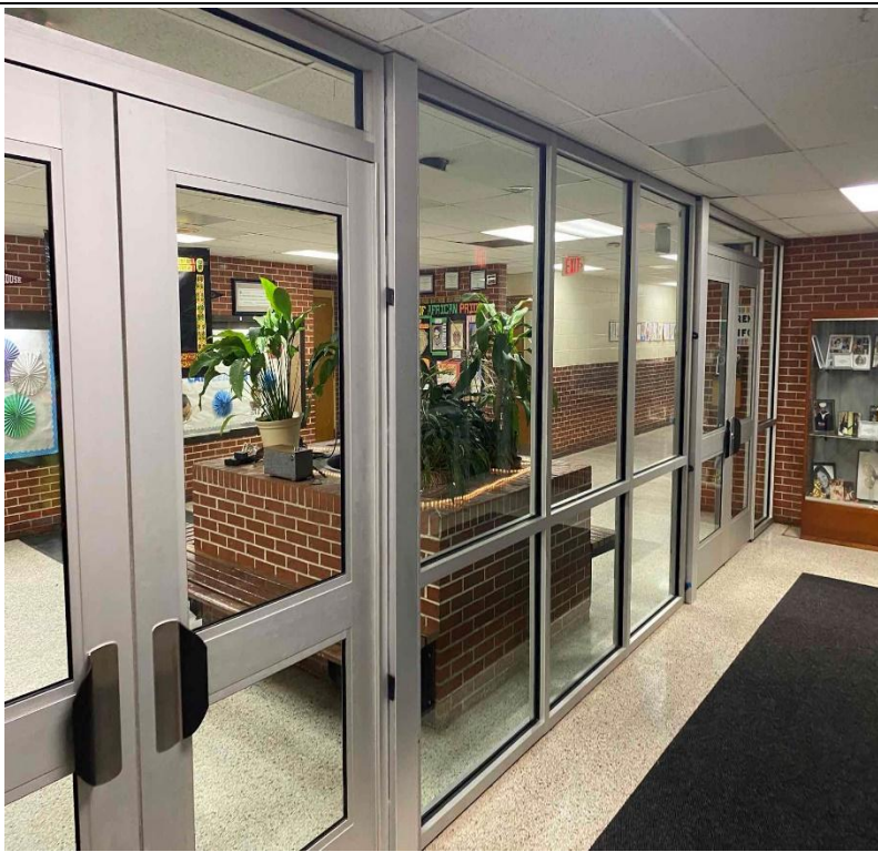
Ballistic Storefront Installation
