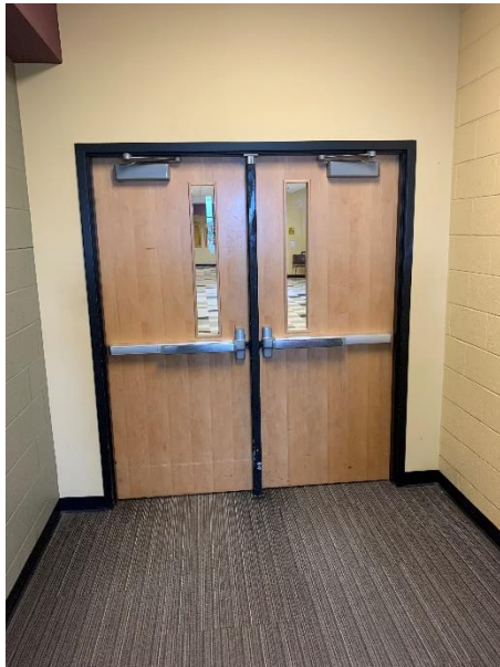
Security Vestibule: Administration Foyer #3
