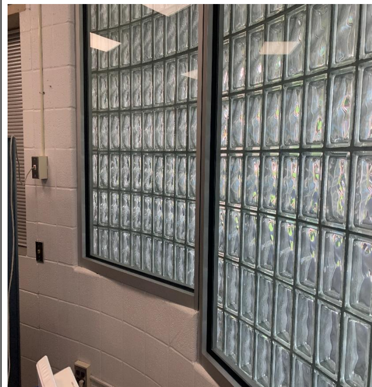
Ballistic Glass in Admin Office Installation
