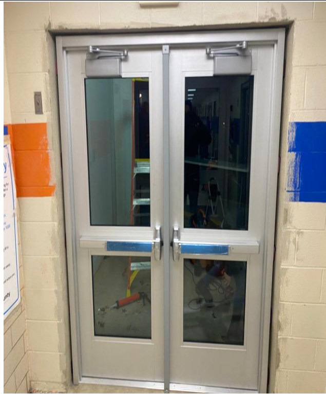
Ballistic Storefront Installation
