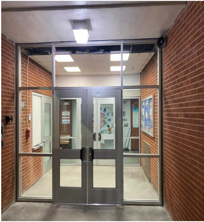
Ballistic Storefront Installation
