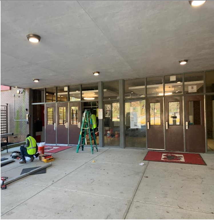
Ballistic Storefront Door Installation
