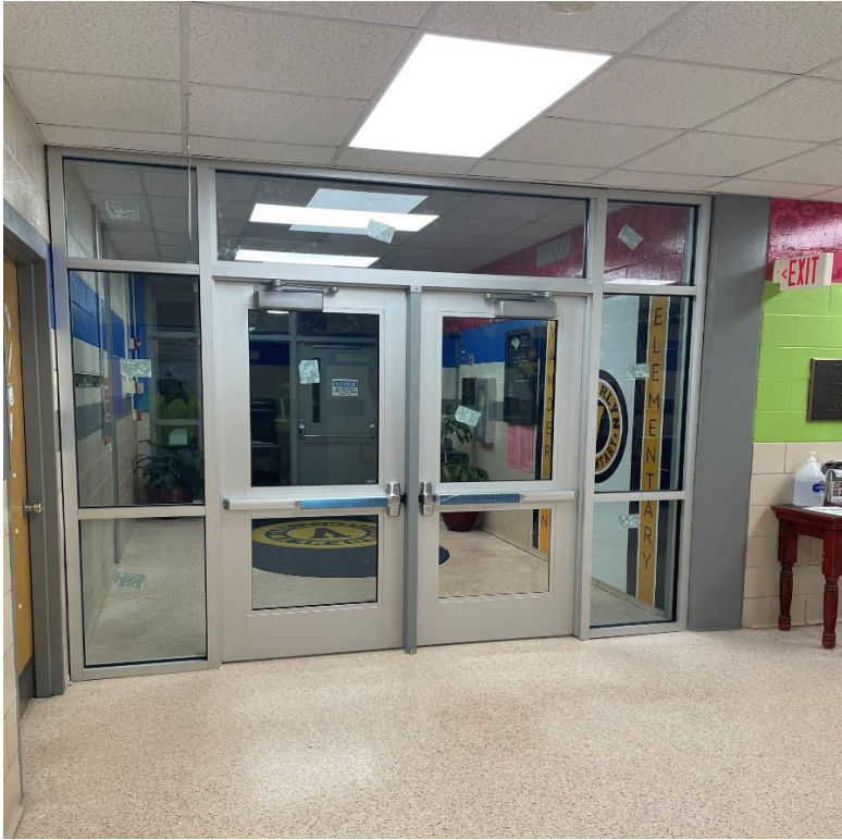
New Interior Ballistic Glass Storefront
