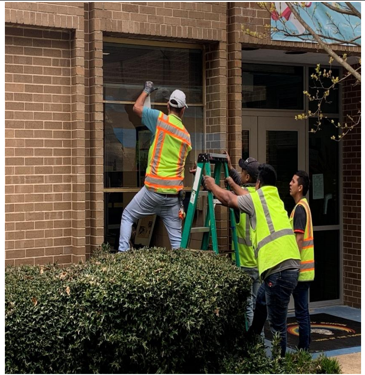
Tampered Glass Window Installation
