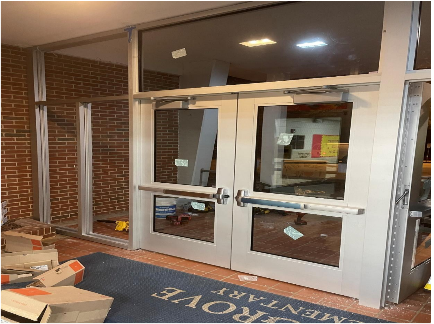
Exterior Storefront Installation
