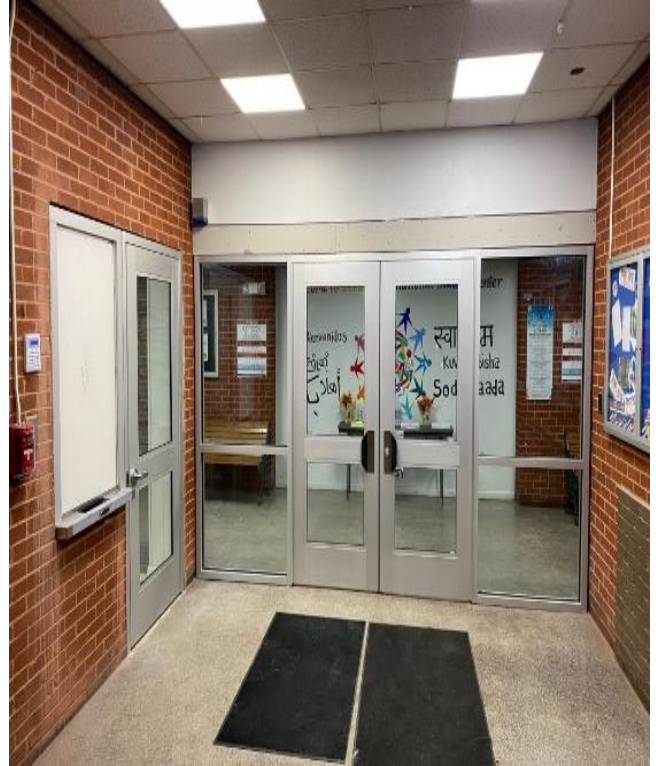
Ballistic Storefront Installation
