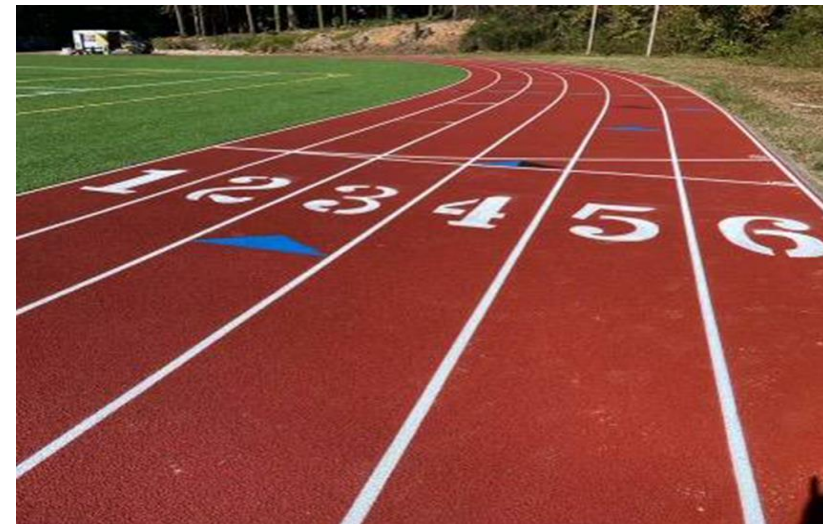
Clarkston HS – Completed PIP Track
