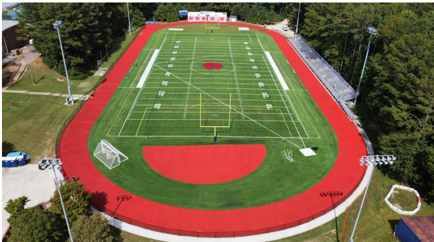
Dunwoody HS – Completed Turf Field and Track
