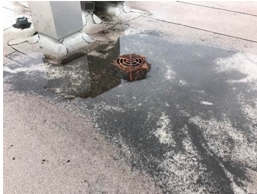
Clean Roof Drains
