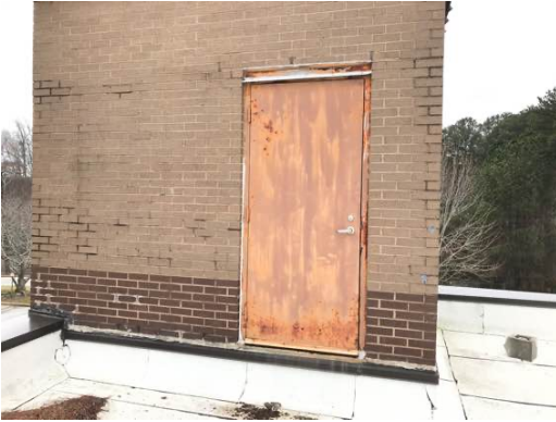
Replace Door On Roof To Bell Tower
