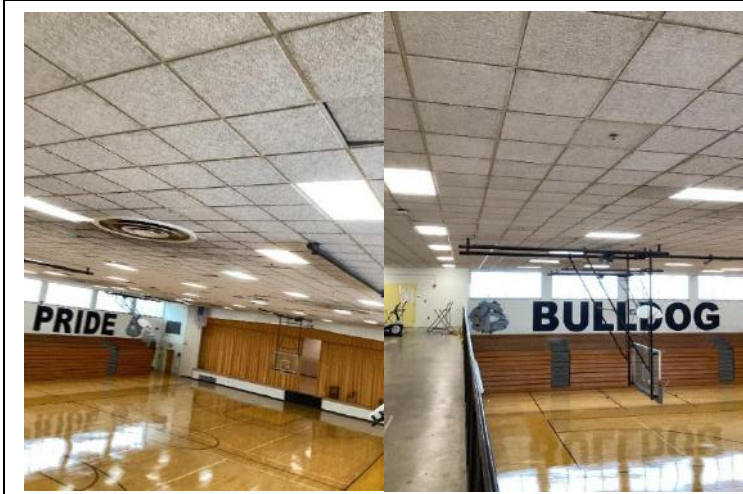
Stage existing conditions
