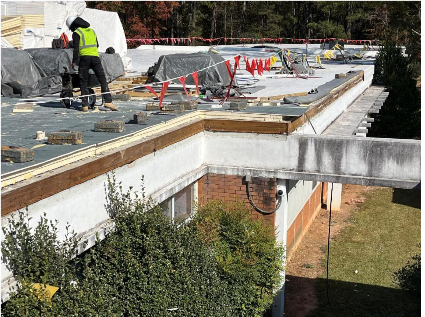
Installation of new roof over admin office.
