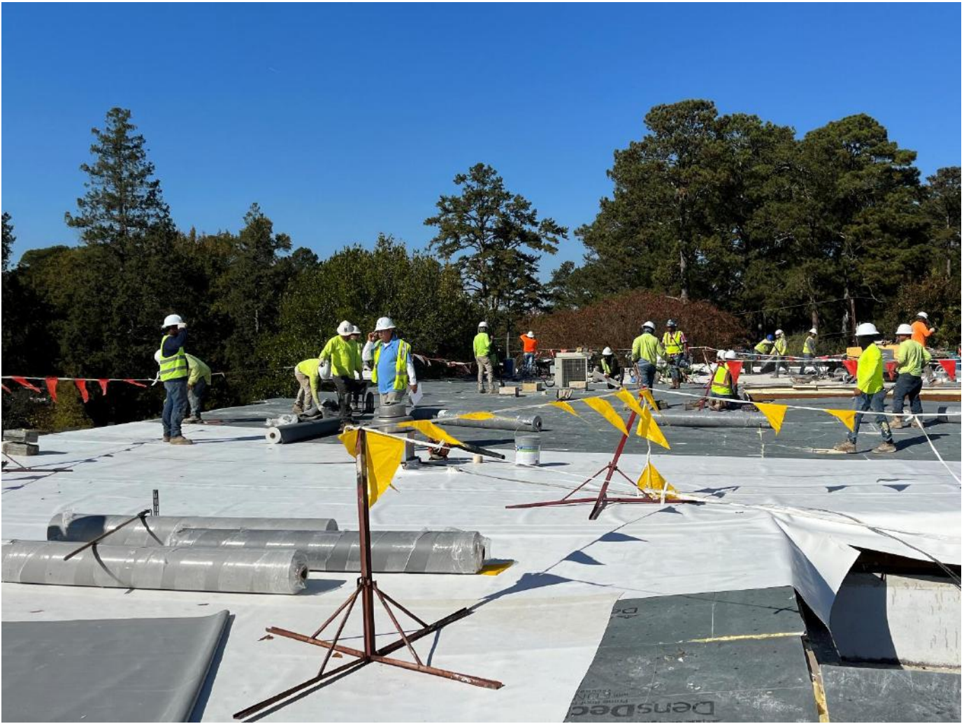
Installation of new roof over classrooms.
