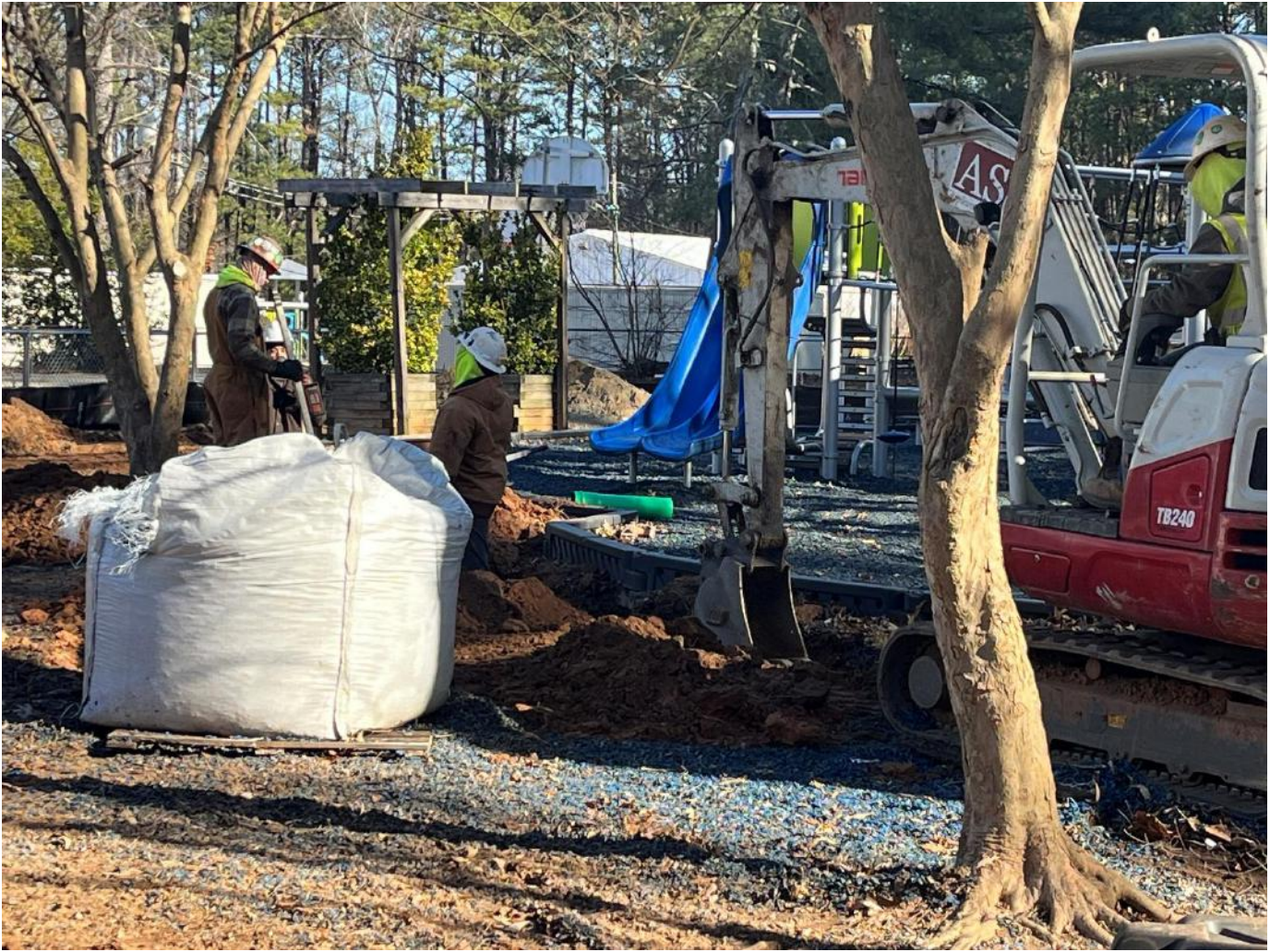
New storm drain pipe installation.
