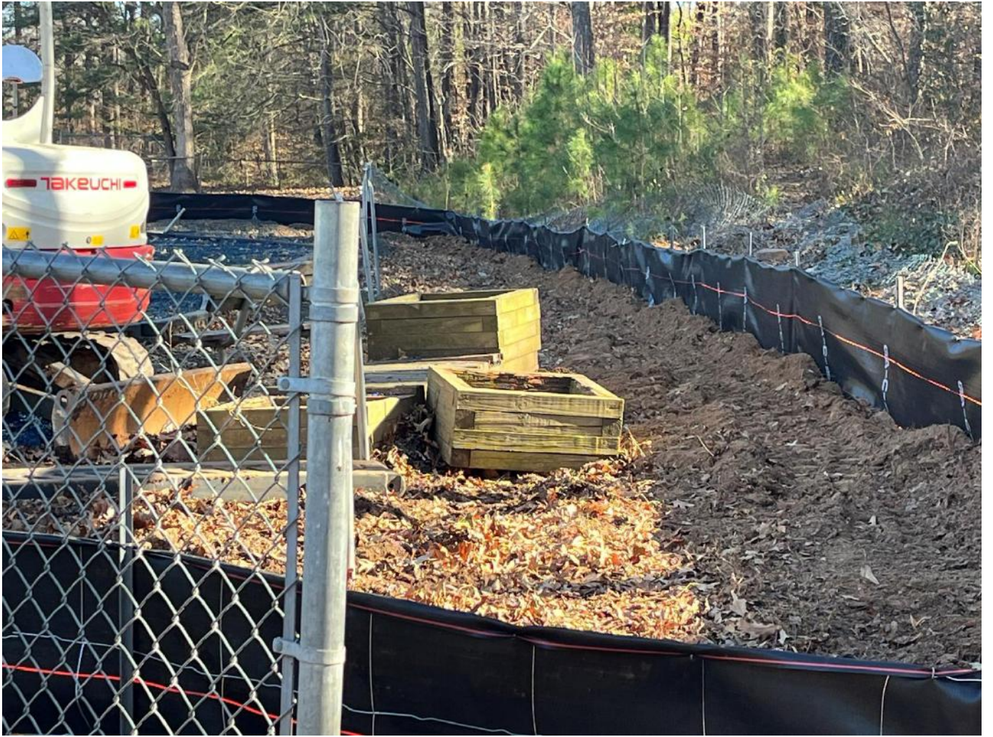
Erosion control installed.
