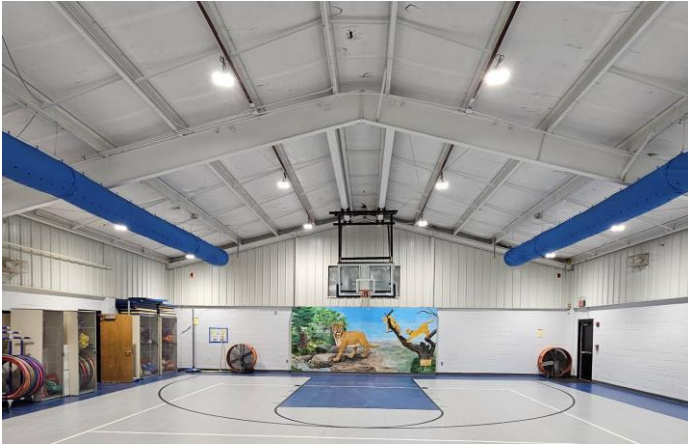
Gym Interior with new Fabric Ducts
