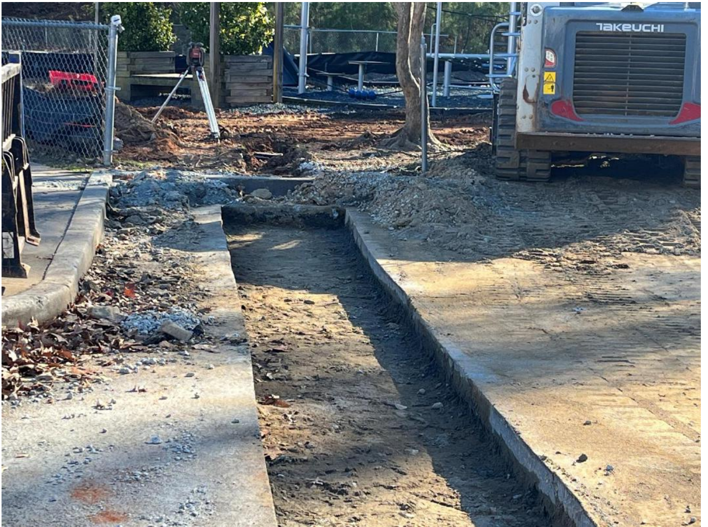
Pipe trench cut to install new storm pipe.
