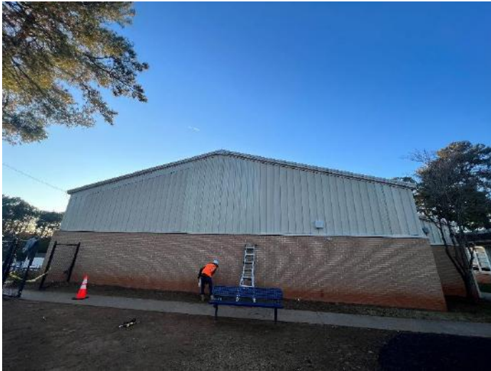
New Exterior Metal Panels
