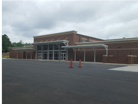
2). South Elevation - May 18, 2016
