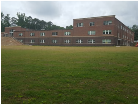
4). East Elevation - May 18, 2016
