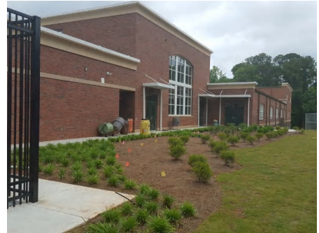
3). East Elevation - May 18, 2016
