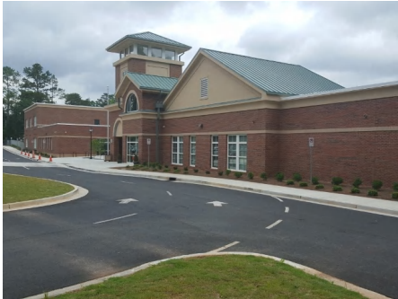
1). West Elevation - May 18, 2016
