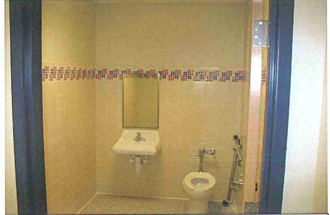
Columbia HS ADA Restroom
