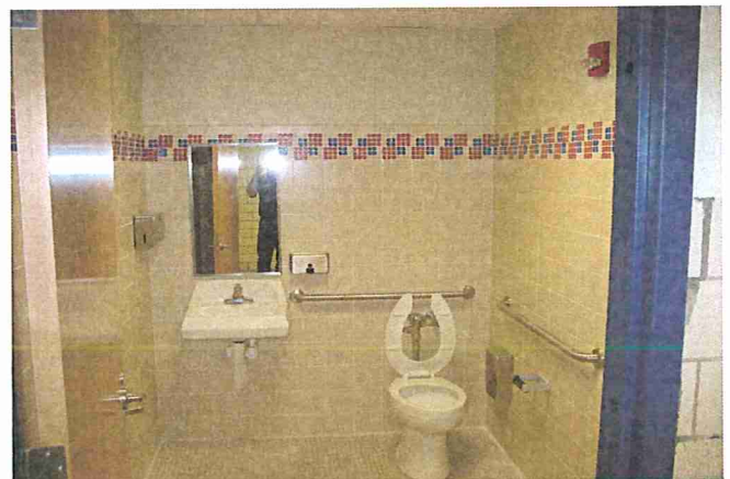
Columbia HS ADA Restroom
