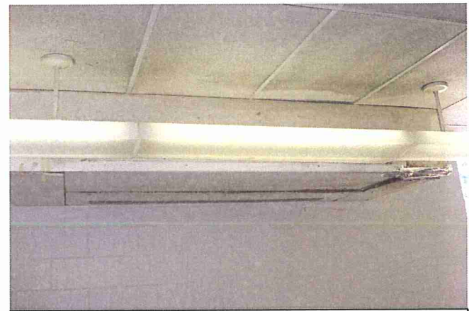
Redan ES Existing Ceiling Grid & Lighting
