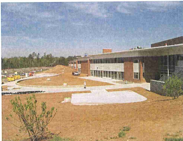
Arabia Mountain HS South Elevation
