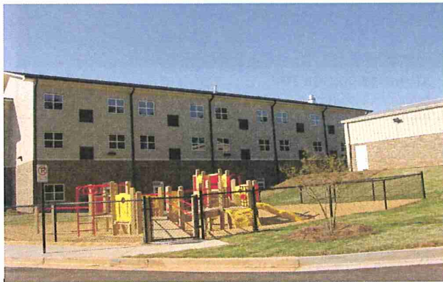
McNair Cluster ES North Classroom Pod & Playground
