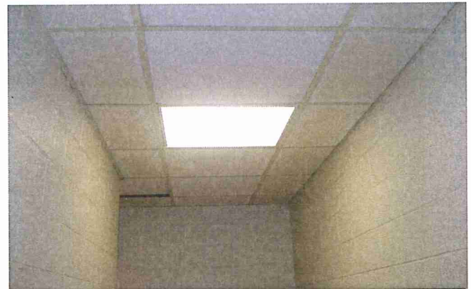
Briar Vista ES Existing Ceiling & Lighting
