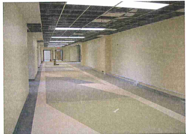
Arabia Mountain HS Interior Corridor
